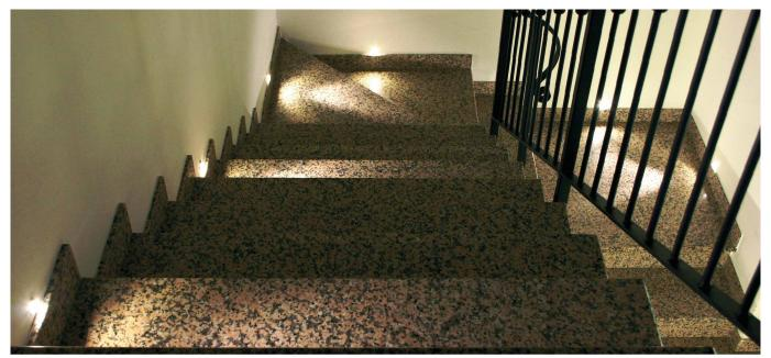
Flush-fitted in polished 304 stainless steel with power LED for accent, decoration, courtesy or step marker lighting. Choice of secondary optics. Can be fitted in the floor, wall or in plasterboard indoors and outdoors. Mounting with formwork.
